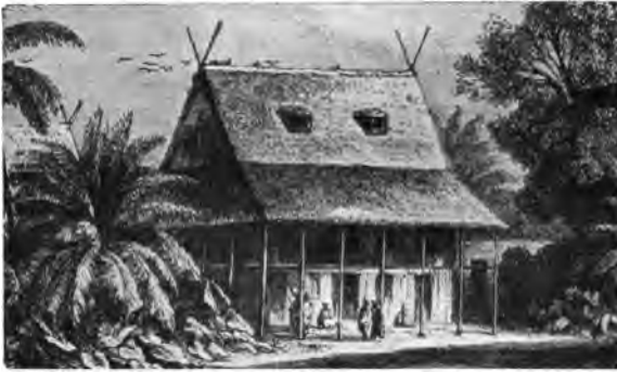
FIG. 16.—Note the forks of this well-constructed four-story house of a Hova chief of Malagassy.
